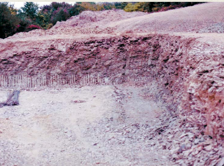
Early stages of construction
